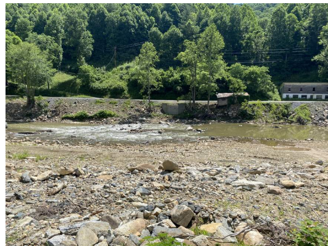
LOOKING EAST FROM END BENT 1
