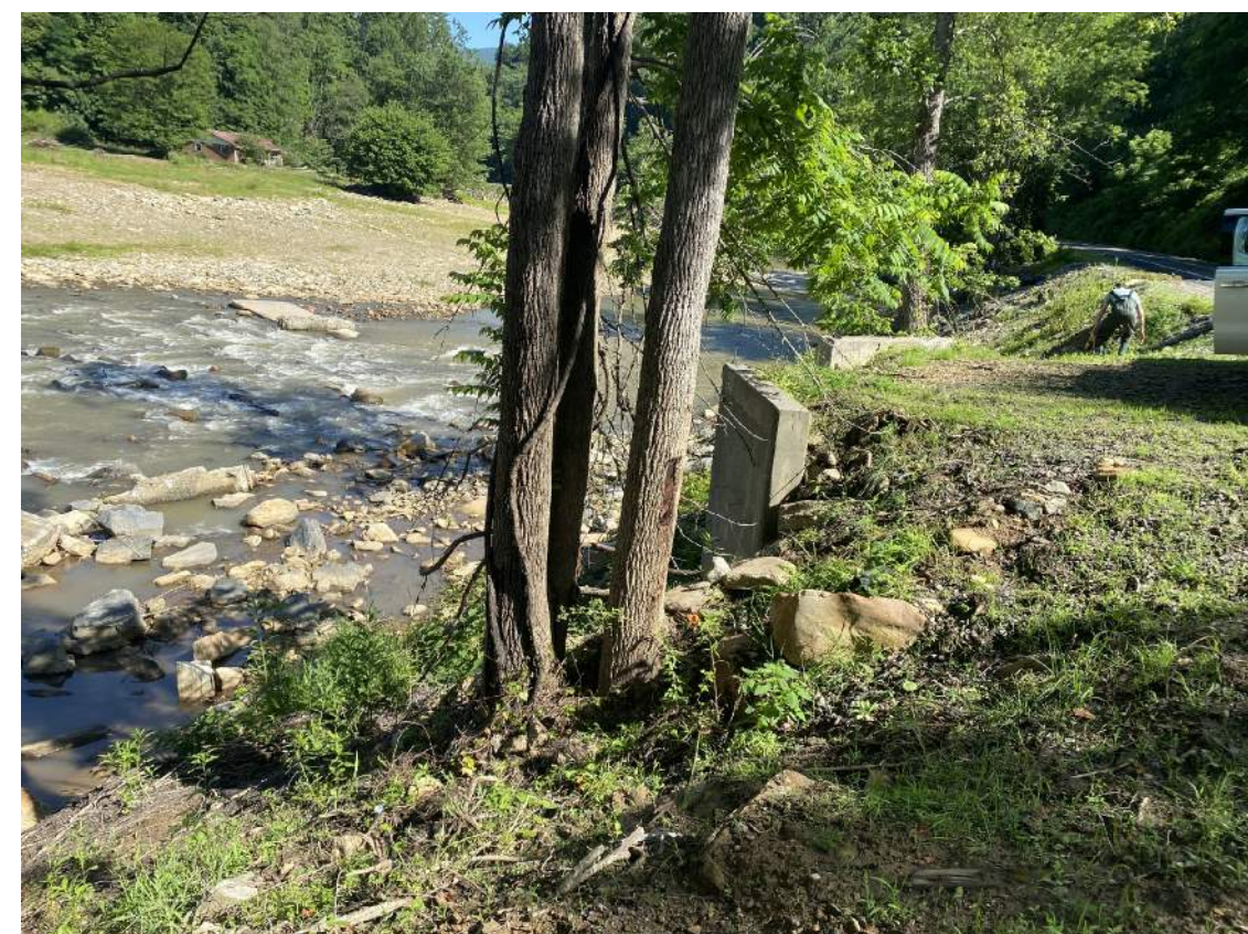
LOOKING NORTH (DOWNSTREAM) AT END BENT 2
