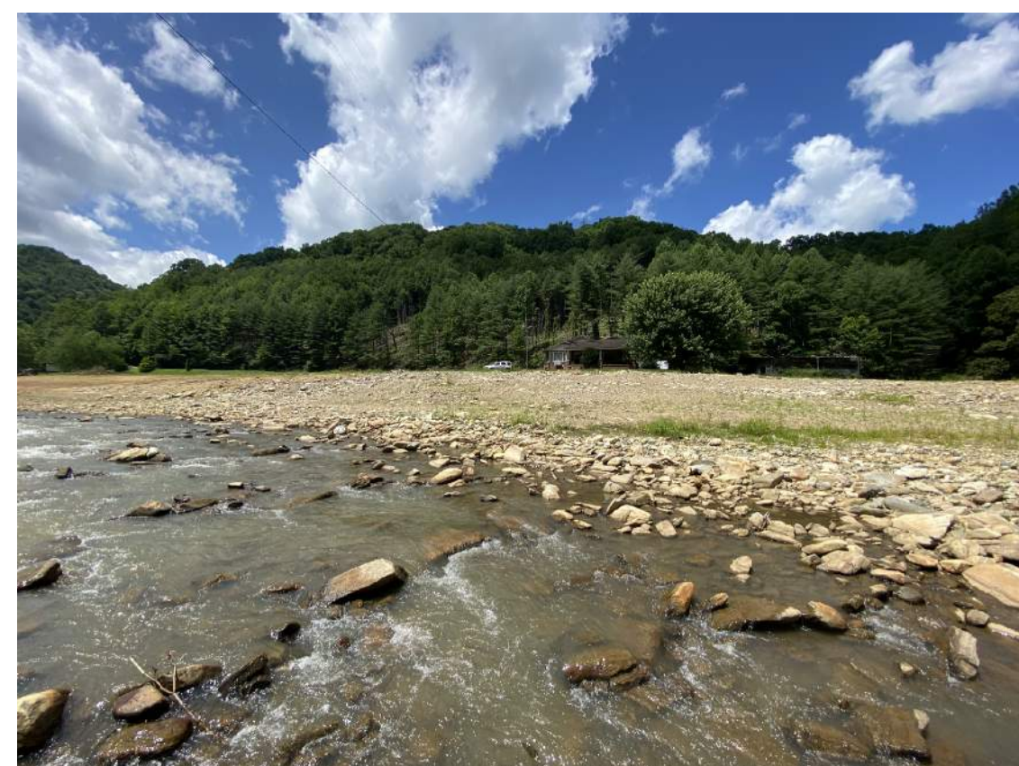
LOOKING UPSTREAM TOWARDS END BENT 1
